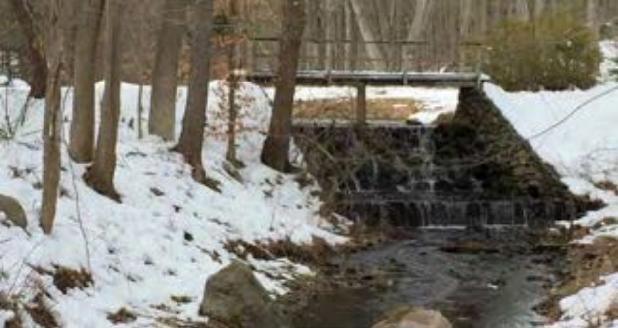
H.J.Halle dam on Salem Road C. Reppert 2018
