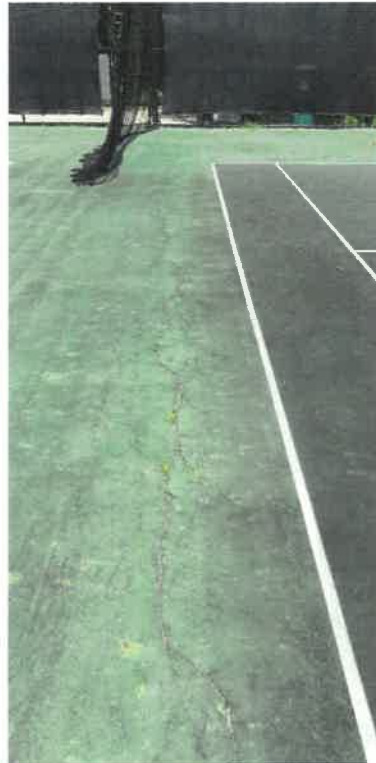
Structural & surface cracks
