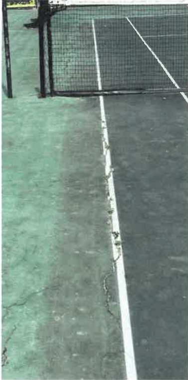
Structural cracks
