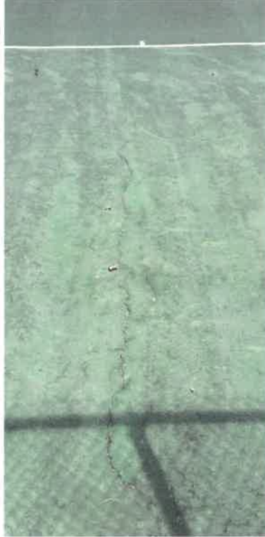
Surface cracks
